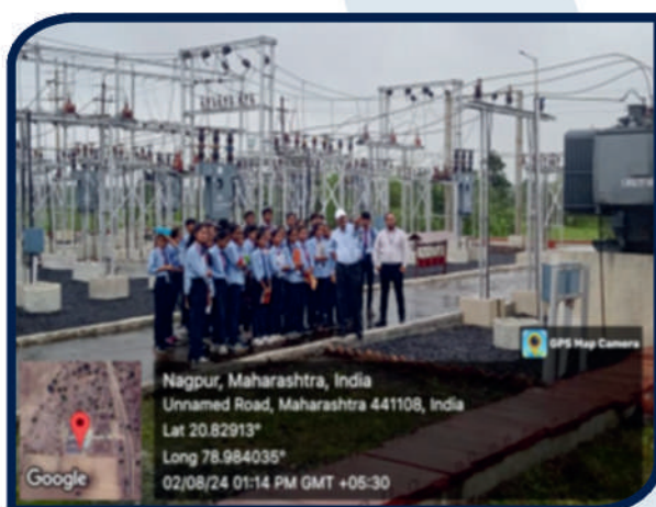
Expert Explaining to the Students & Faculty during visit at MSEDCL 33kV/11kV Substation at Alagondi, Butibori, Nagpur
